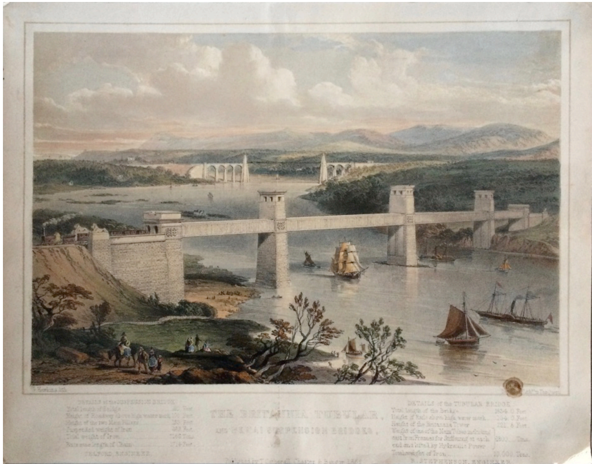
7. [G. HAWKINS]. BRITANNIA BRIDGE. "Britannia Tubular and Menai Suspension Bridges", showing train and shipping, by and after G. Hawkins. Hand-Coloured Lithograph, heightened with gum arabic, showing train and shipping, by Day & Son, mark on imprint to right , Published T. Catherall, Chester & Bangor, 1852. 9.5in x 12.25in £65 Stephenson's Tubular Bridge over the Menai Straits was opened in 1850. Telford's road bridge in the background was built between 1820 and 1826.
